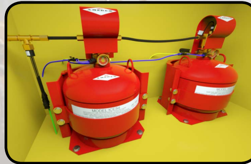
Dry - ICE Cylinders
